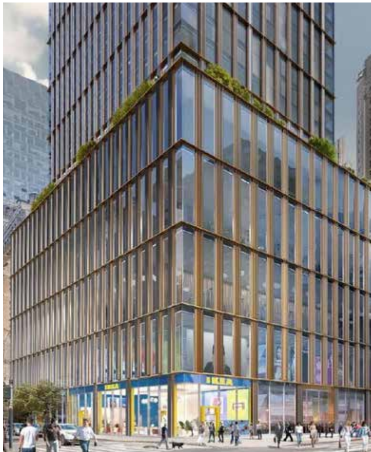
W 46th Street entrance. Image from Excell.
